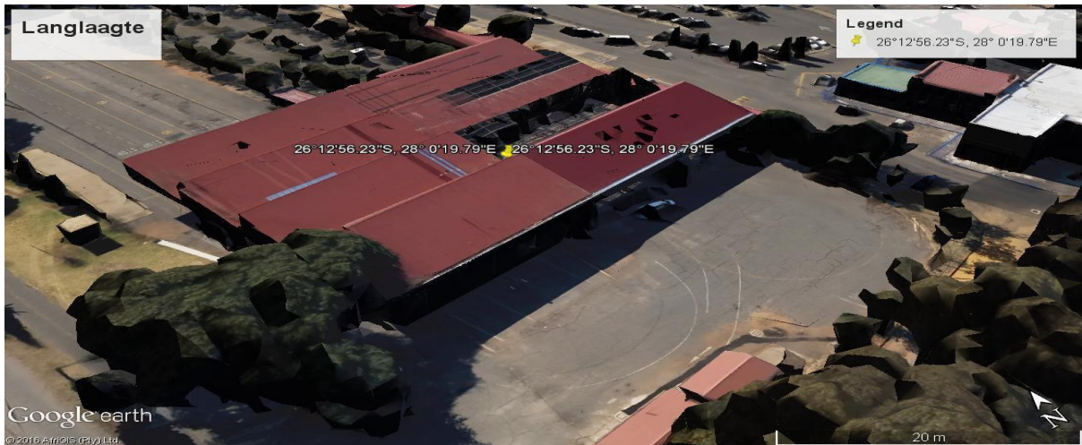
Figure 4.5: Langlaagte roof space from GEP
