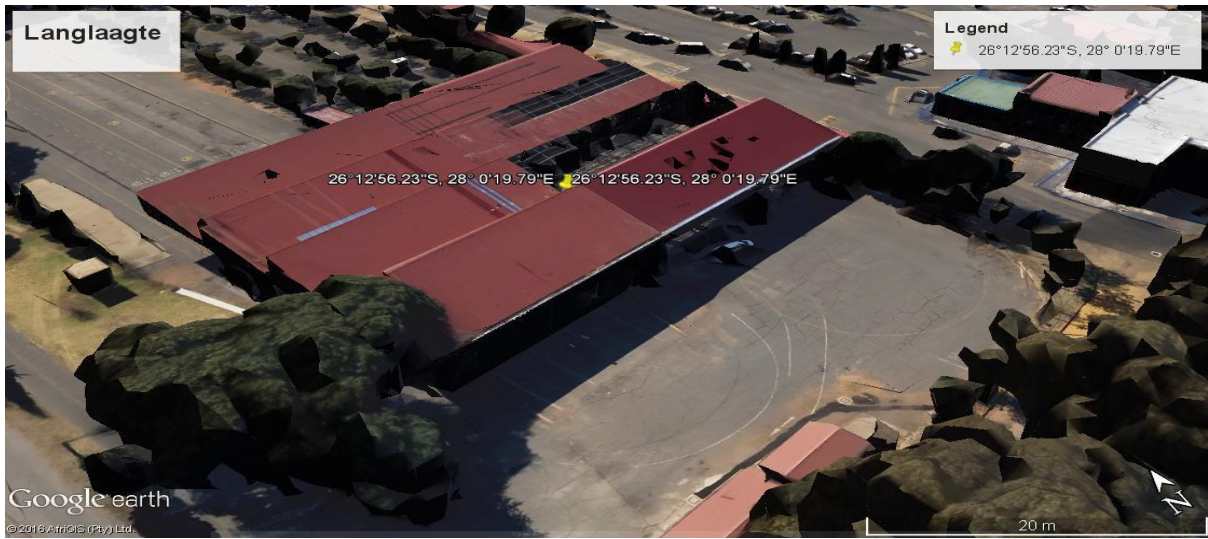
Figure 3.1: Langlaagte roof space from GEP
